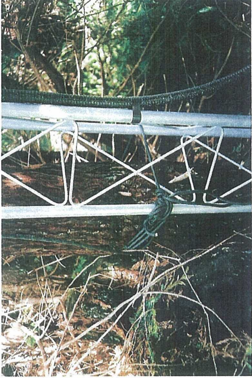
#3 KZCC Tower Tied to tree trunk Tower has no foundation or grounding
