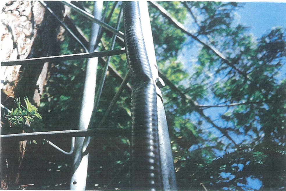
#7 KZCC damaged/ defective transmission line—Note significant kink
