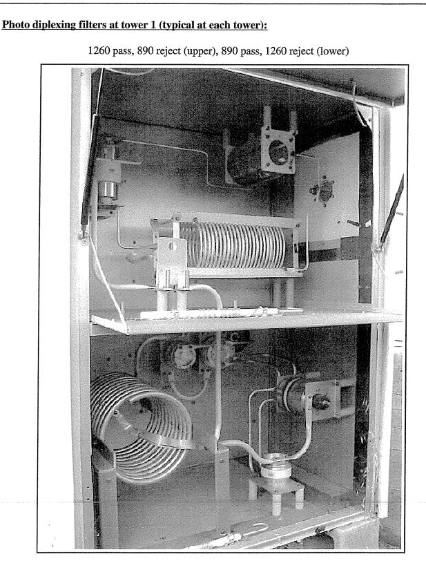
The KXTK tower feed loops through the upper compartment, from the right. The J plug in the center is where KLFF joins the KXTK feed to the tower which exits to the left. This is the same equipment which has been in use at KXTK-KLFF for over a decade. No changes were made.
