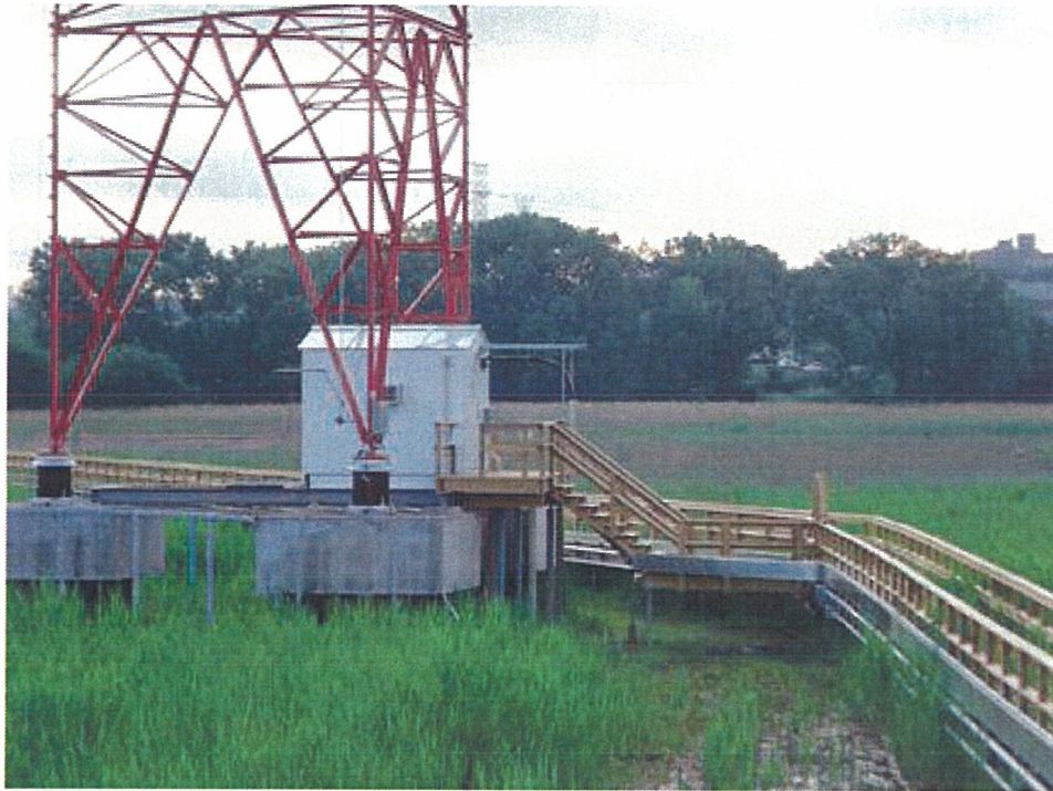
Above: The base of Tower 1, the center tower, as seen from Tower 2
