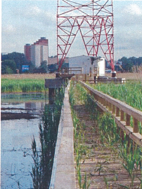
Left Above The base of Tower 2 from the main boardwalk. Note the heavy growth of marsh grass between the planks.
