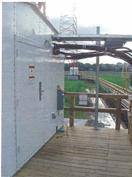
Above: Tower 2 porch and shelter entrance looking east toward Tower 1.
