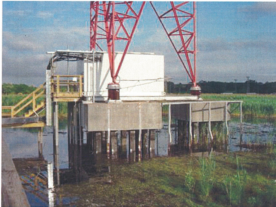
This view of Tower 2 looking towards the west shows the basic configuration of all three towers. The major difference is that Tower 2 has the larger shelter to accommodate the phasor.
